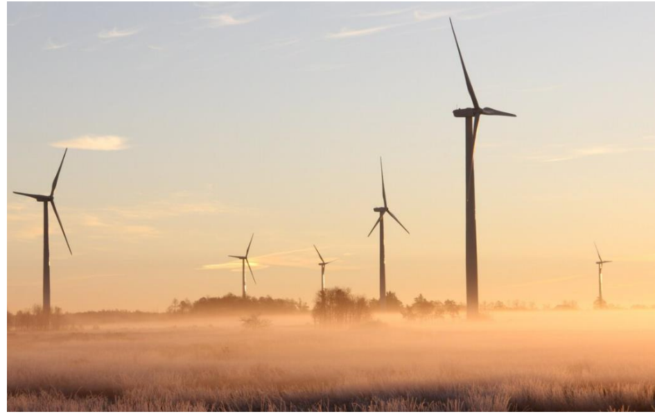
Wind Farm. Source: RENEW
